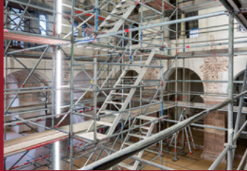
Baufortschritte in Corvey
